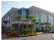
The Timely touch enhances major office buildings across the country.
